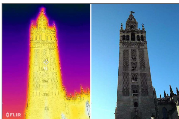
Figure 8: thermographic analysis of the north façade of the Giralda bell tower. We can see, on the left, the photograph taken by a thermographic camera and, on the right, the same photograph taken by a photographic camera. We can see, on the left, the photograph taken by a thermographic camera and, on the right, the same photograph taken by a photographic camera (photographs by the author).
