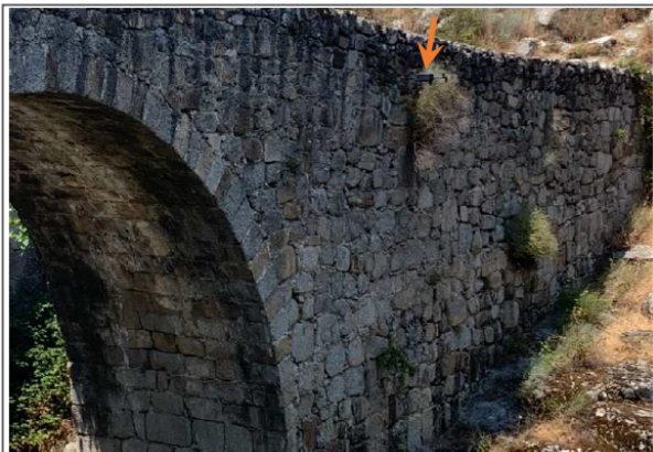
Figure 5: Drone equipped with a thermal imaging camera, approaching a medieval bridge (Puente del Grajal) for inspection (photograph by the autor).
