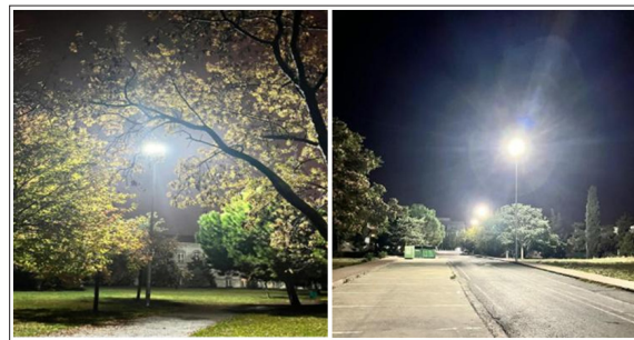
Figure 2: Examples of Luminaires Commonly Used on Campus
