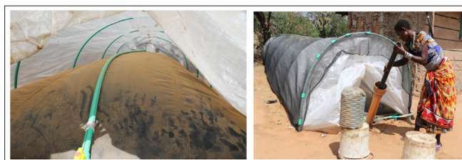
Figure 5: Showing a biogas digester unit that provides enough energy to meet the needs of a household with up to 12 people. Biogas use in slaughterhouses was observed to be limited.
