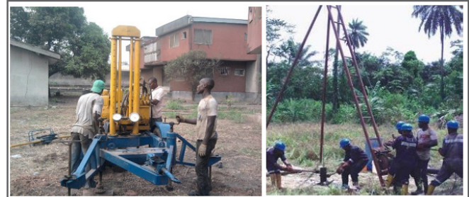
Figure 4: (a) 10 tons cone penetration testing, (b) boring and SPT
