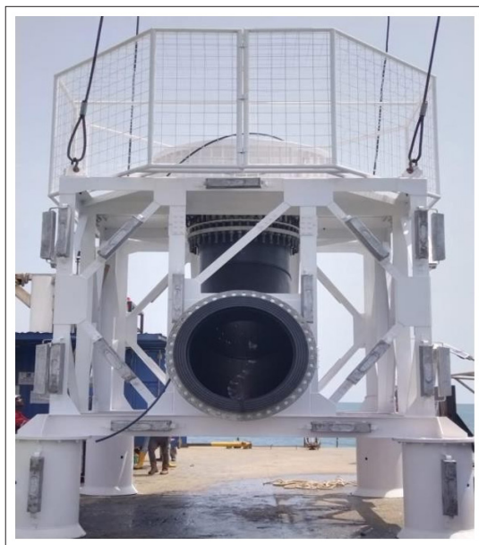
Photo 1: Seawater intake head structure
