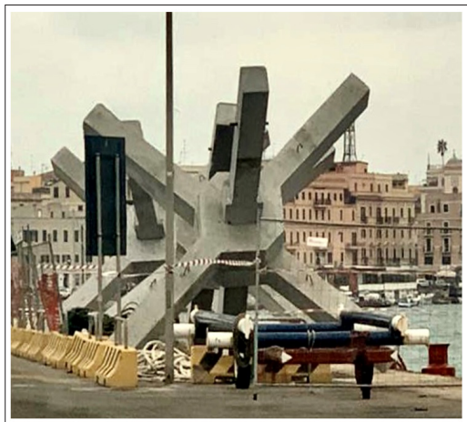
Figure 1: Example of anti-trawl tripod module. Sizing of a single tripod
