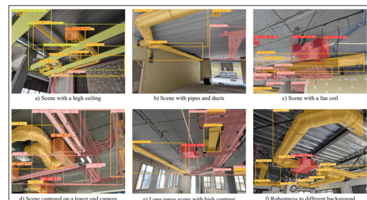
Figure 8: Qualitative examples of successful instance segmentation results using the YOLOv8 model (Mixed-20%) on diverse real-world indoor construction scenes. (a) Scene with a high ceiling, showcasing detection of ducts and radiant panels. (b) Scene demonstrating differentiation between pipes and ducts. (c) Accurate detection of multiple fan coil units amidst clutter. (d) Performance on an image captured with a lower-end camera. (e) Long range scene with high contrast. (f) Robustness to different background.
