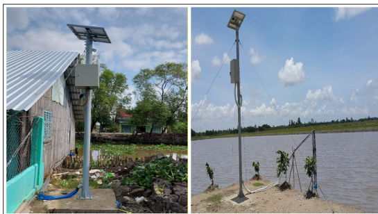
Figure 6: Environmental monitoring stations at Ray Moi canal and in rice field areas for rice - shrimp farming systems
